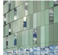
2. PREFABRICATED EXTERIOR CLADDING METAL PANEL SYSTEM - THREE TONE CUSTOM COLOR PAINT ON METAL PANELS
