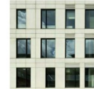
4. PUNCHED WINDOW GLASS SYSTEM WITH ANCHORING
