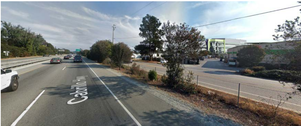
View of the project from southbound travel lane of Highway 1.
